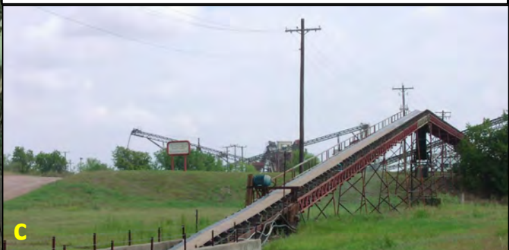
View of the existing conveyor belt system (c) to be used to transport finished material from the plant to the existing Fordyce dock (d).
