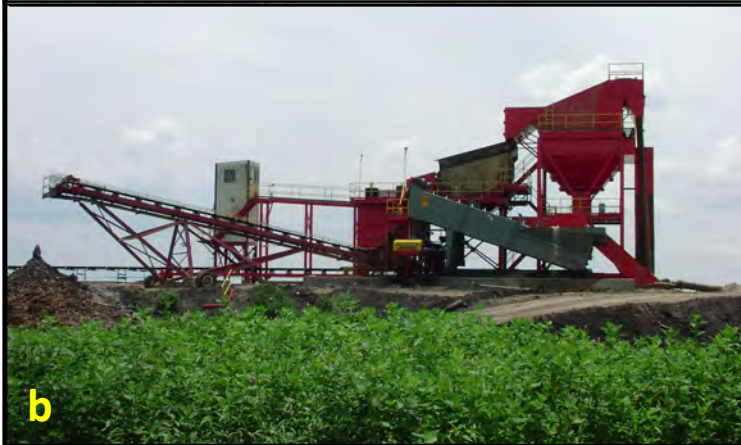
Representative view of a dewatering/de-sanding plant (b).
