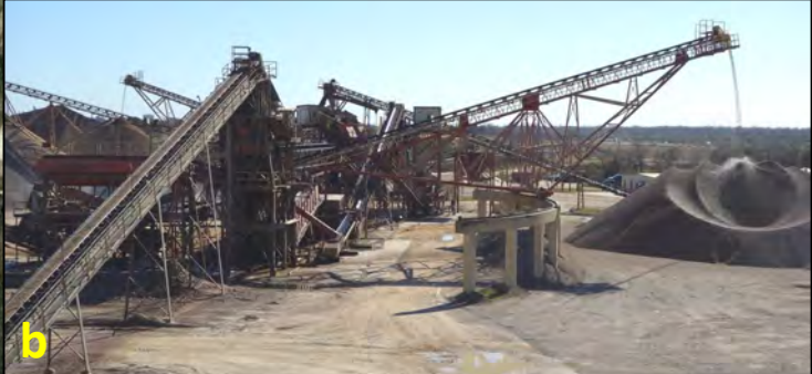
View of the existing processing plant (b) where the material will be washed, separated, sized, and crushed as necessary to meet customer specifications.
