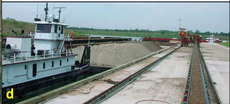
View of the Fordyce dock (d) at the north end of the Victoria barge canal, where finished material will be loaded onto customer barges using existing gantry.
